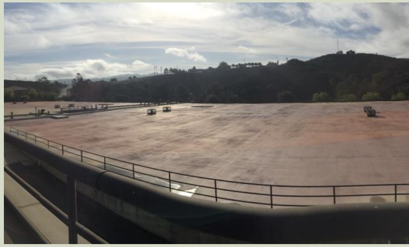
Clearwell Reservoirs (8 MG)
