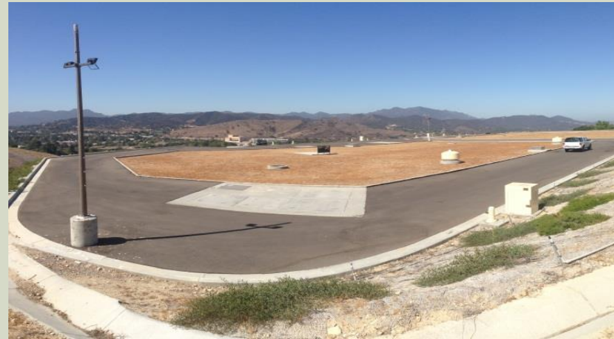
Thousand Oaks Reservoir (7 MG)
