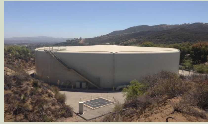
Newbury Park Reservoir (3.8 MG)
