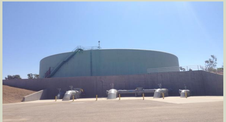
Grimes Canyon Reservoir (5 MG)
