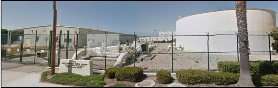
Port Hueneme Brackish Water Facility
