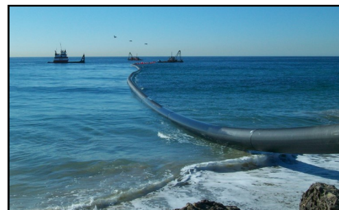
Ocean Outfall Construction
