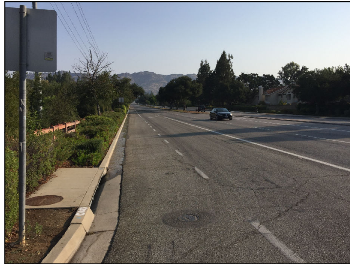
c. CMWD pipeline alignment at Rockfield Street, facing north
