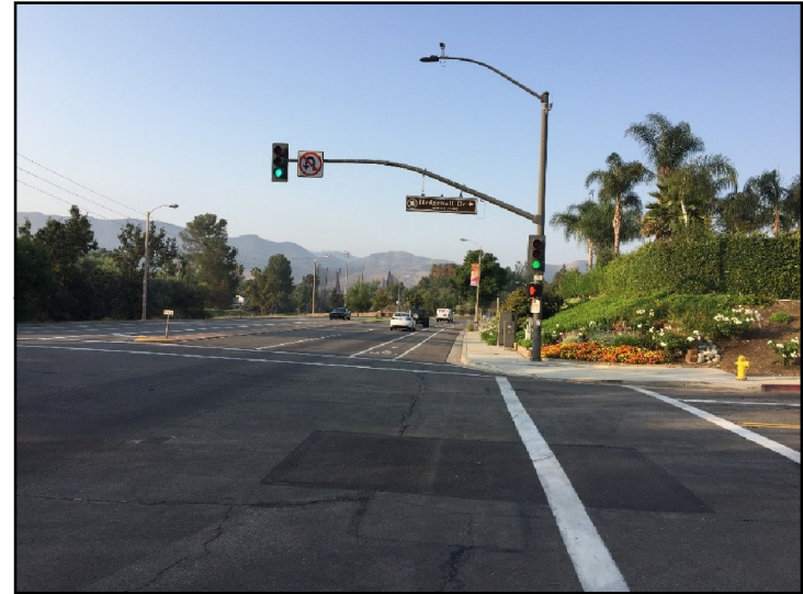
b. South Interconnection pipeline alignment at Hedgewall Drive, facing south
