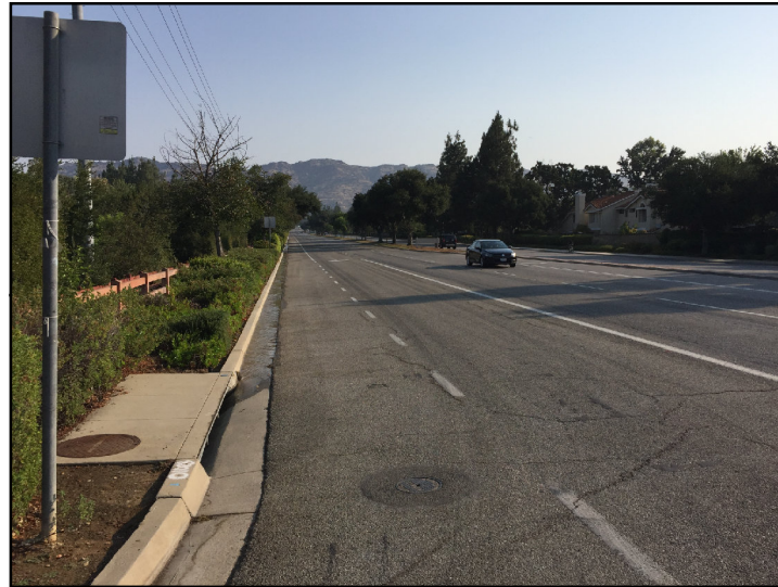
c. North Interconnection pipeline alignment at Rockfield Street, facing north
